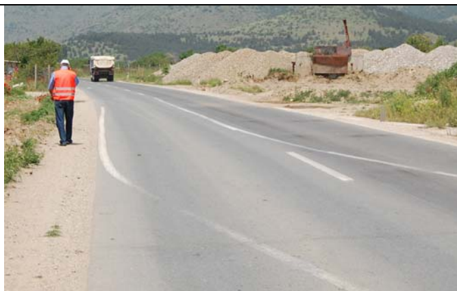
Figure 2.14. Marking in bad condition, old "phantom" marking
