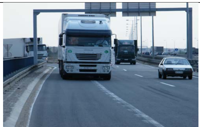
Figure 2.4. Weaving lane to narrow for large vehicles
