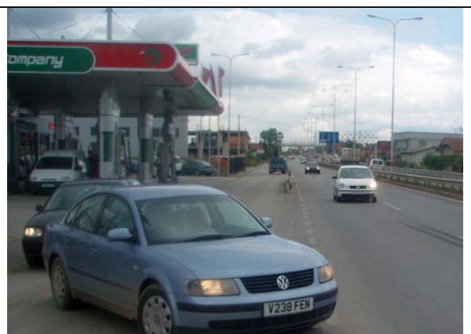
Figure 2.2. Express road with parallel service road but direct access from a petrol station to the main carriageway
