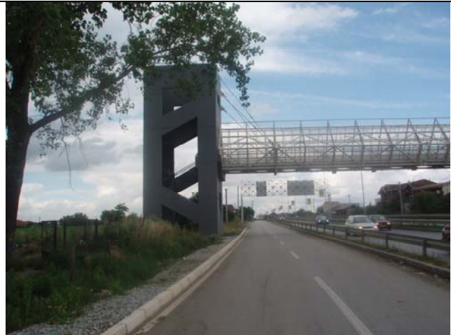
Figure 2.10. Modern pedestrian bridge crossing an express road with adjacent service roads, but lack of connection to guide the pedestrians
