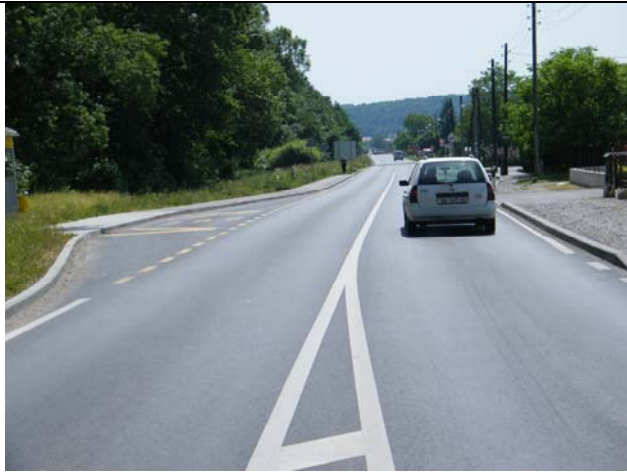
Figure 2.9. Bus-stop with lay-by, lack of crossing facility and connecting footpath
