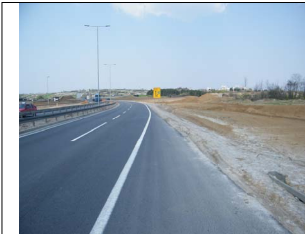
Figure 2.5. Curve sequence with small radii after a long stretched section is not visible
