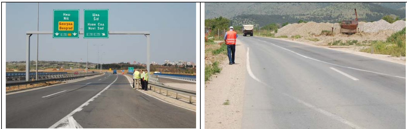
Figure 2.13. Insufficient directional signing solution, misleading marking
