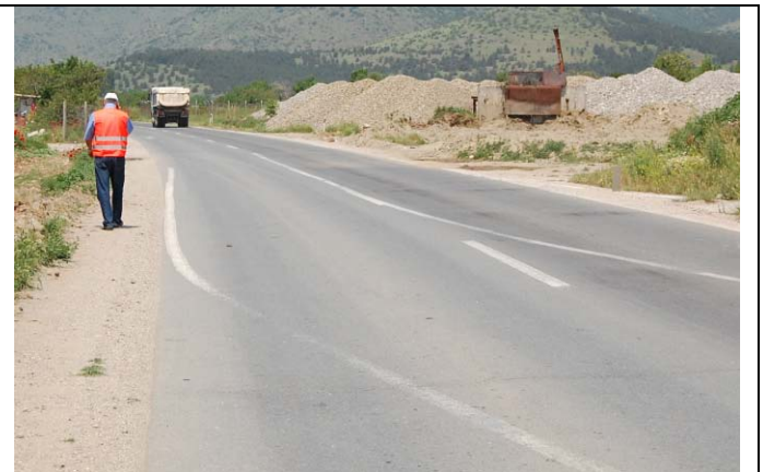
Figure 2.14. Marking in bad condition, old "phantom" marking
