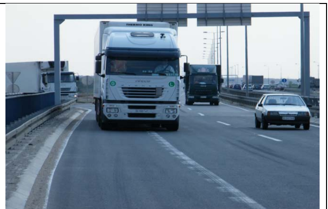
Figure 2.4. Weaving lane too narrow for large vehicles
