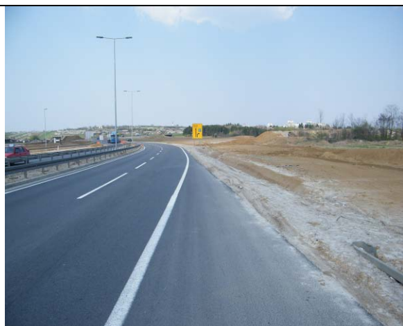
Figure 2.5. Curve sequence with small radii after a long stretched section is not visible
