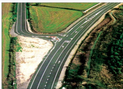
Transformation from a Y intersection to a T intersection.
